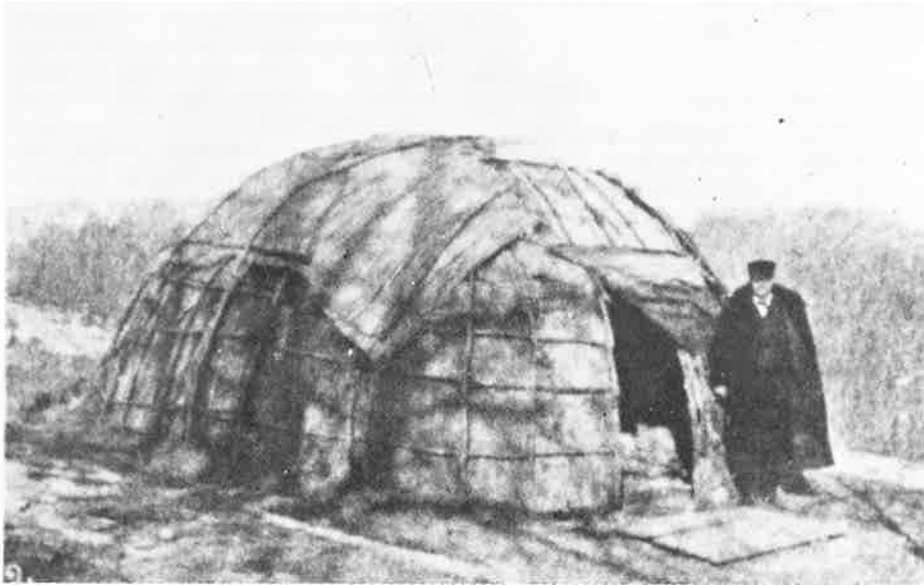
Typical Winnebago Reed Matting Lodge - Historic Period. Photographed in Nebraska (Courtesy Smithsonian Institute.)
